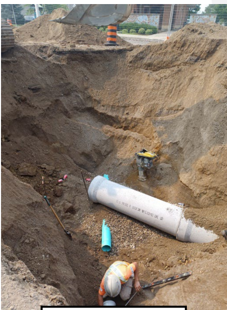
New concrete Sanitary sewer
